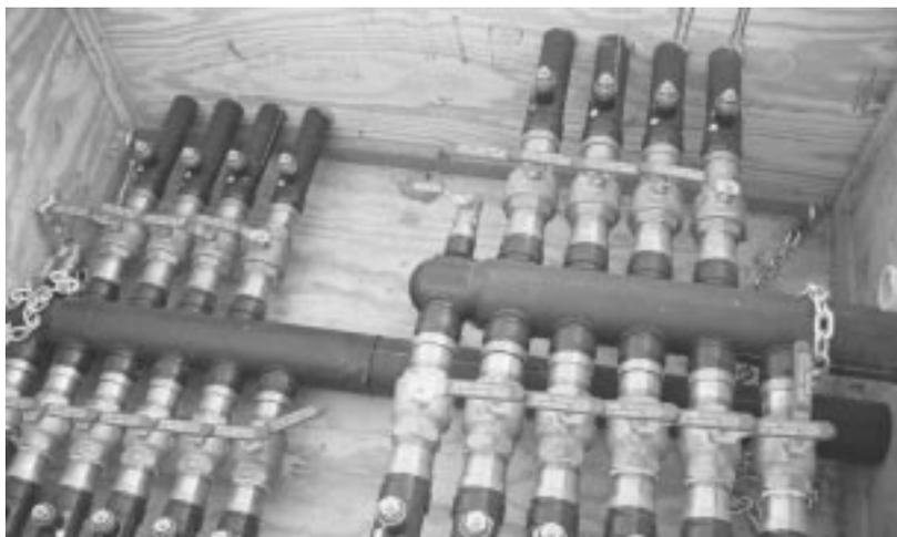
*The two header assemblies for the shallow heat exchangers will be used to control and monitor the system.*
