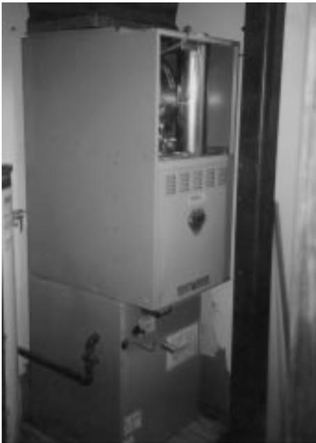
The new furnace and coil were installed in the same location as the old unit. An additional air return vent and grill were installed in the living room to accommodate the higher capacity air handler.
