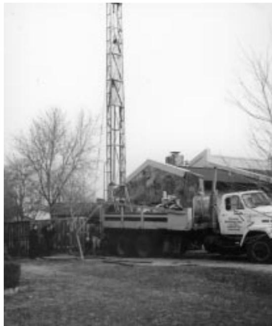
*Four 200 foot bore holes were drilled using an air rotary rig in order to avoid a mud clean-up problem. The loops were spaced 12 feet apart to eliminate the thermal influence from one loop to another.*
