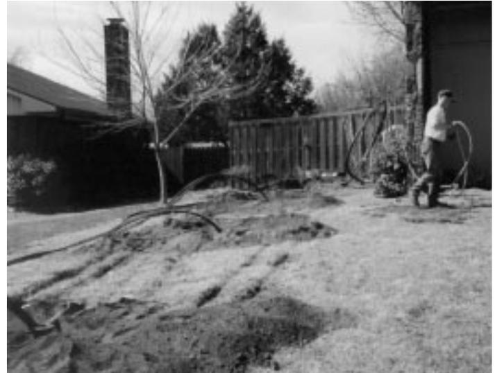
*Before each of the four loops were installed in the boreholes, they were filled with water, checked for cuts and pressured tested for leaks. The loops were then heat fused and connected to the supply and return headers and placed in a four foot deep trench up to the outside unit.*
